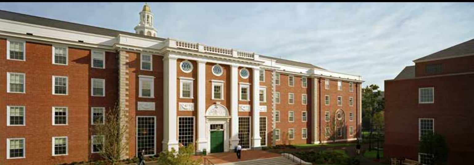
NEW SOUTH FACADE
